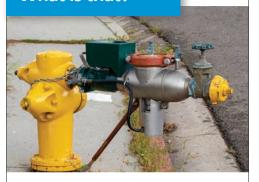
Have you ever seen this device on a water meter, and wondered -- what is that? It's a temporary water meter. We use these devices when customers need short-term water service -- at a construction site, for example -- so that we can track and bill for the water they use.
