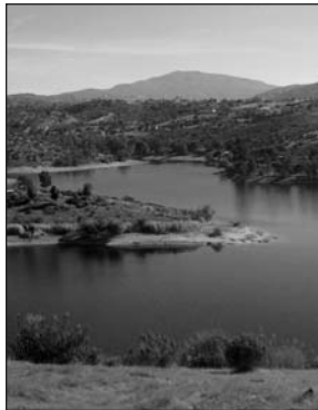
Lake Jennings is the District's reservoir. It has a 9,790 acre-foot capacity.
